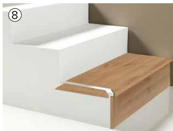
Cut the stair nose to the measure of the step and finish it off. Miter cut the right side (A) to fit it to the other stair nose. Crosscut the left side to miter (B). Clean the groove, then fix it to the step with silicone.
