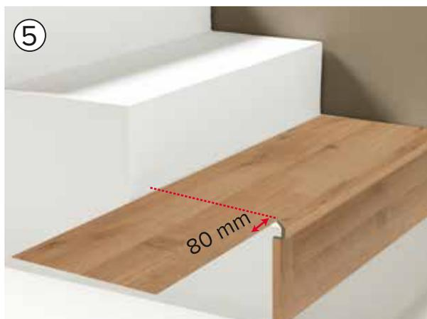
Measure the length of the step, subtracting again the measure of the stair nose (80 mm) and cut the plank at both sides to the measure, make sure to clean both the tongue and the groove.
