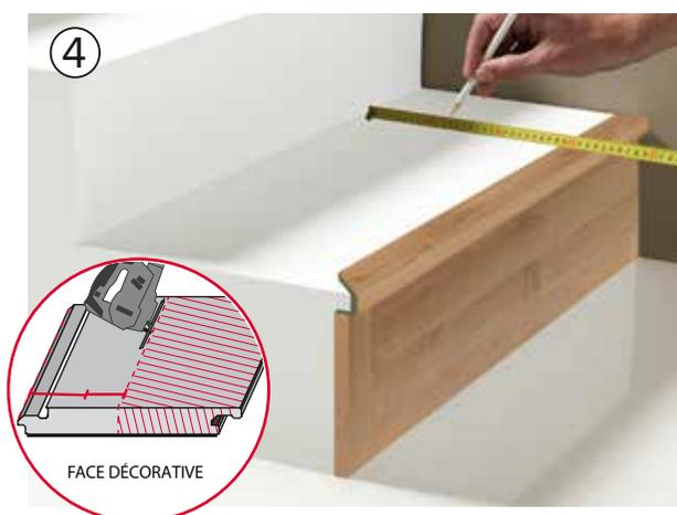
Provisionally, place the stair nose and measure the distance (riser) from the front to the profile. Next, cut the plank facing the decorative side down. Note that you should add 2mm to the previously measured distance, counting from the side of the tongue.
