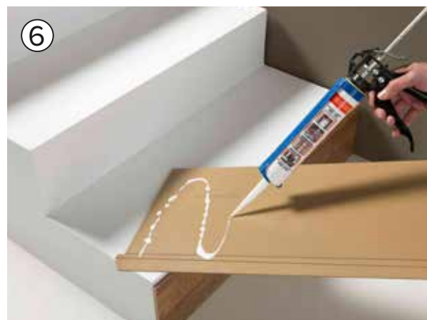
Glue both parts together (plank and stair nose) and fix it to the step with silicone.
